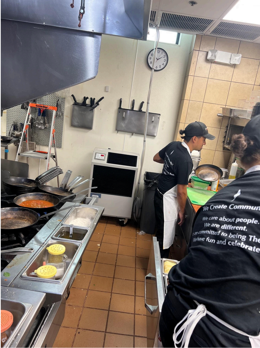
Two hot cooks in East Dundee, IL when the heat was excruciating in the summer of 2023. We installed a couple of Oceanaire OWC1811 water cooled units in the kitchen area and another one located at the entrance to the restaurant. Portable water cooled are the alternative when an air-cooled unit is not an option. Restaurants are common applications for spot-coolers. Our Climate Control team is always on their toes to answer your call when the phone rings. Dropping what you are doing afterhours and weekends is not uncommon, since customer service is always Rent AC's top priority.
